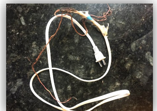
Extension cord involved in an office fire at W&M.
